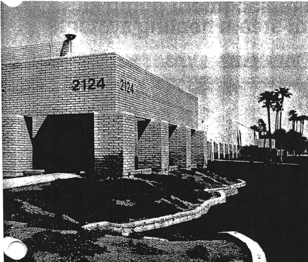
The eutectic thermal storage system will cool the Arizona Public Service Company 120,000-square-foot Deer Valley Data Center in Phoenix. The system will reduce peak demand by 210 kilowatts.
