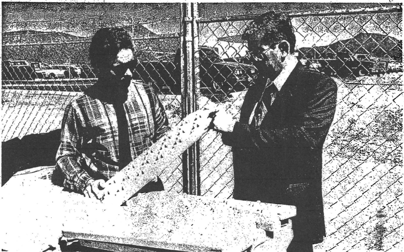
Approximately 45,000 sealed plastic containers, each filled with 1.1 gallons of a special eutectic salt solution, were installed inside the buried concrete tank to form the heart of the latest thermal storage system installed by the utility as a demonstration project for its commercial customers.
